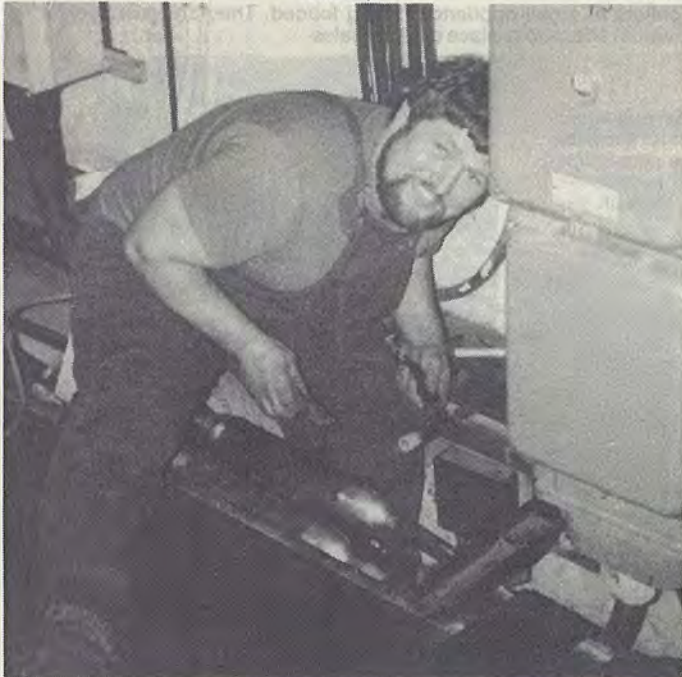
Craftsman Paul Taylor completes a cable joint at the Ferodo factory
