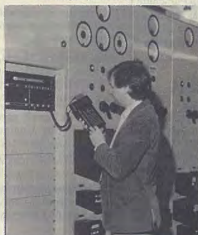
Below, 1st engineer John Hampson checks on the MANWEB-invented micro-processor relay. The "small black box" will eventually replace all the relay equipment shown in the larger picture to the left
